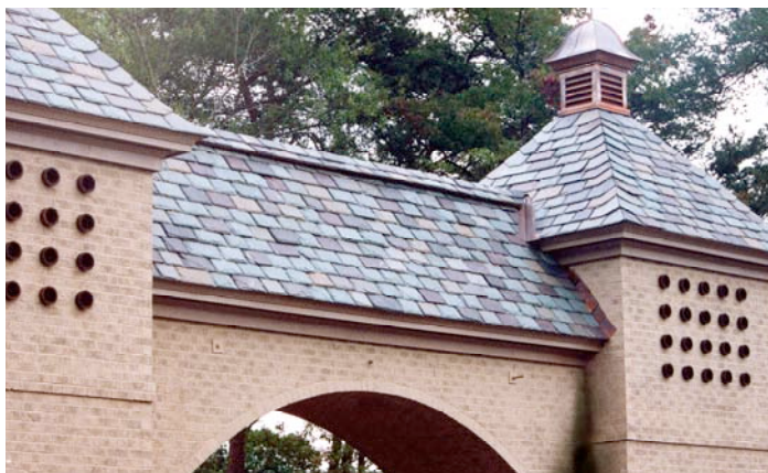
TOP: Semi-weathering slates complement a stone façade, with random widths for a traditional application. Photo courtesy of Evergreen Slate.
