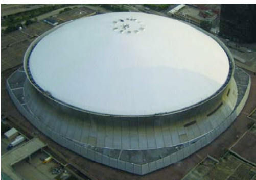
LEFT: In 2005, after Hurricane Katrina destroyed the roof, the New Orleans Superdome was repaired in record time, with a fluid-applied coating system and foam roof. Photo courtesy of BaySystems North America
